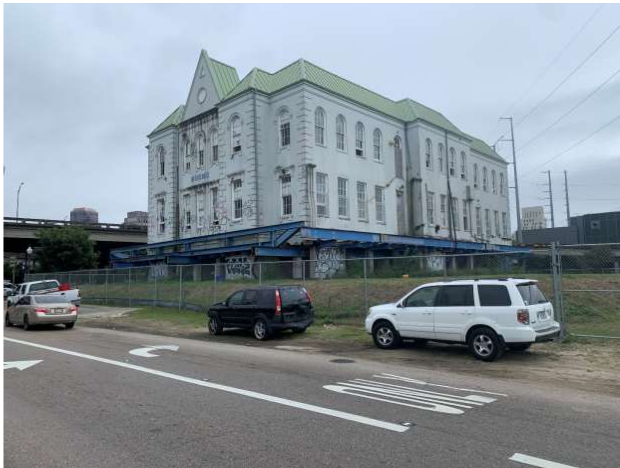
Front and side view of the subject property
