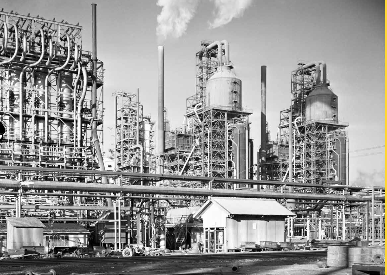
The three cat crackers of the Baton Rouge refinery. Cumene plant in the foreground. Photo by Edwin and Louise Roskam, 1943. Pictured at left: Aboard the tug Bertha towing a 7,000 barrel barge of crude oil from Bayou de Glaise to Baton Rouge. Whiskey Bay Pilot Channel. K.J. Marioneaux, pilot. I.J. Marioneaux, pilot. Lowering the pipeline hose to load up with crude oil. Photo by Arnold Eagle, 1946. Louisiana images from the Standard Oil (NJ) Collection, Archives and Special Collections, University of Louisville.
