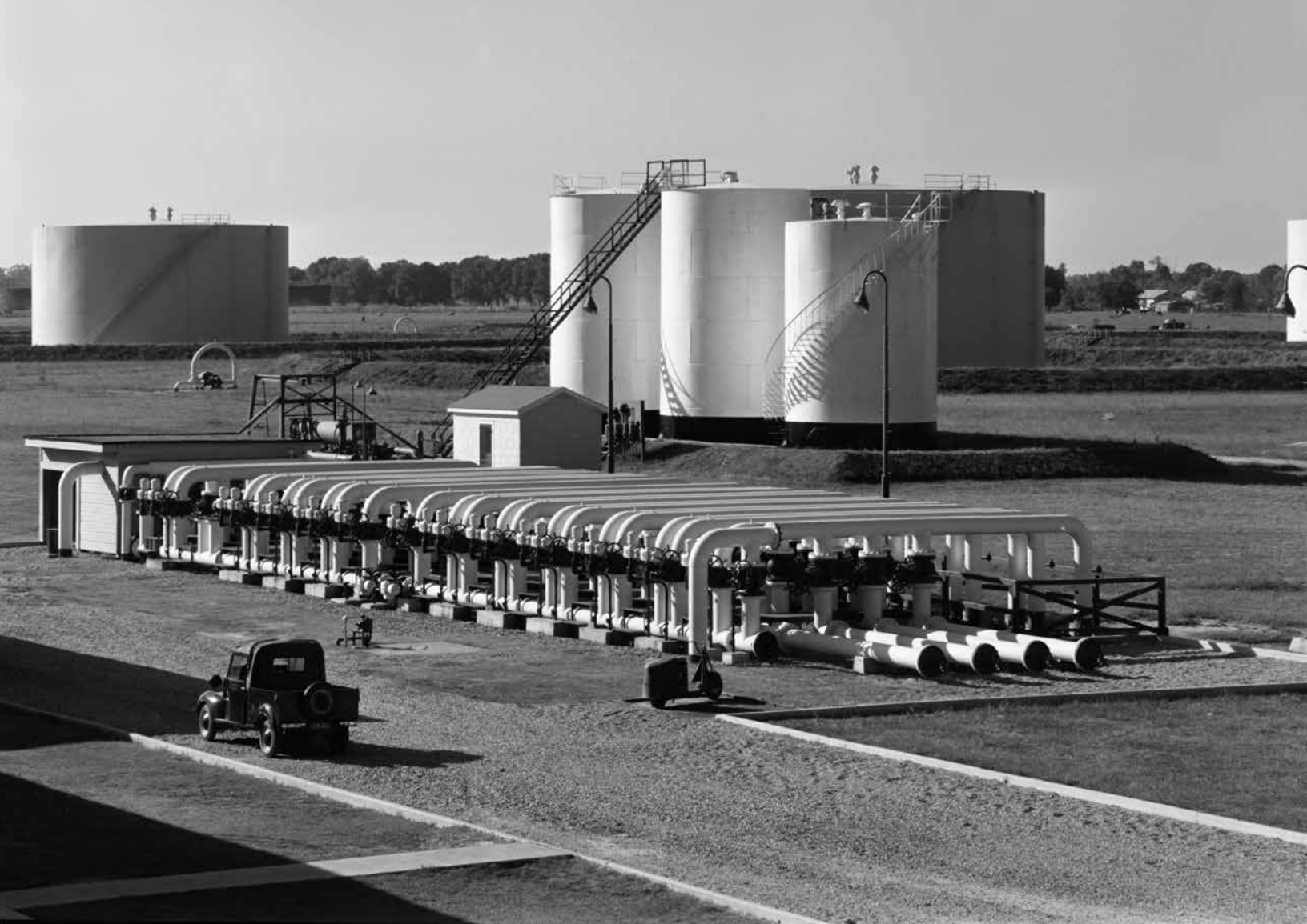
Baton Rouge tank farm of Plantation Pipe Line Company. In foreground is manifold, which controls flow to and from 48 tanks on farm. Photo by Sol Libsohn, 1944. Louisiana images from the Standard Oil (NJ) Collection, Archives and Special Collections, University of Louisville.
